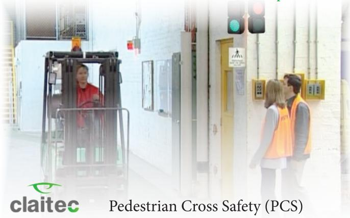
The Pedestrian Cross Safety (PCS) solution is a system of traffic lights that indicates the presence of pedestrians crossing to forklift drivers.
